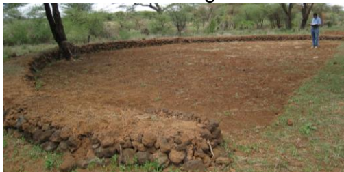
Figure 10. Semi-circular bund constructed in Chumvi Yare, Isiolo district of Kenya.
