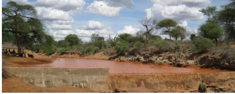
Figure 46: Reinforced concrete dam in Mwingi, Kenya.
